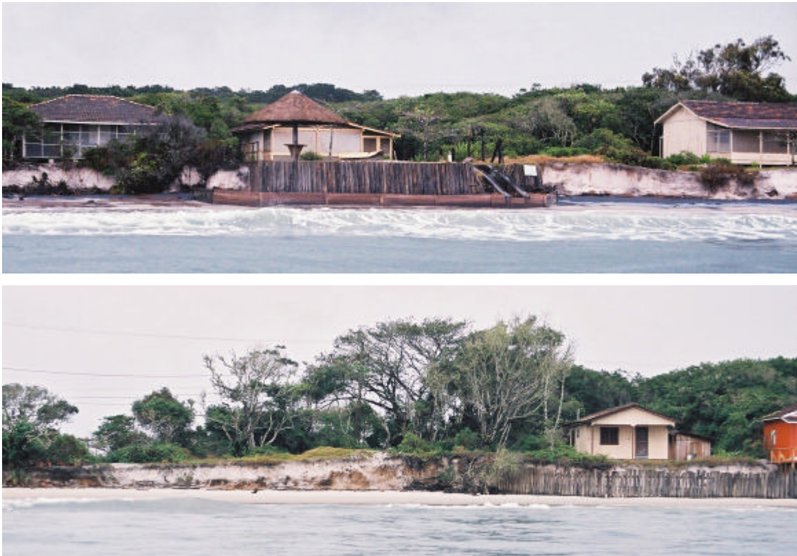
Figure 37: Coastal erosion at Fortaleza beach induced by changes in the wave refraction pattern.
